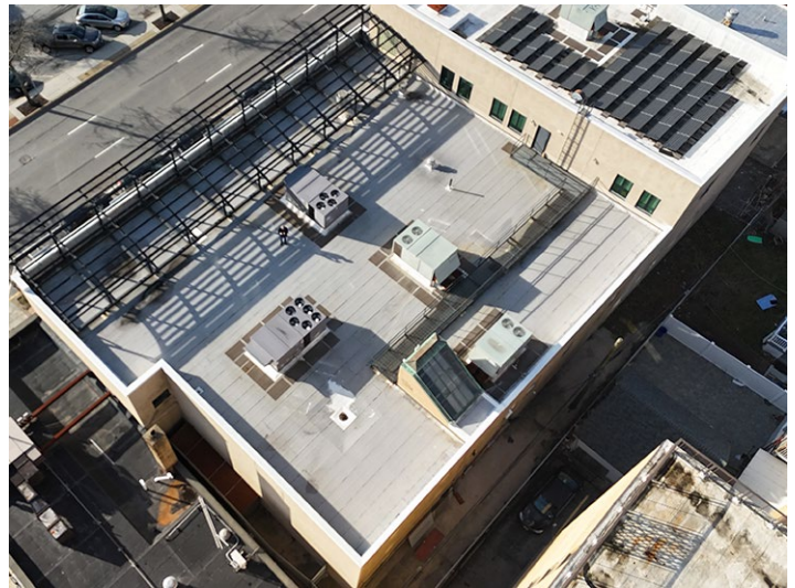
Roof – Lower & Upper
