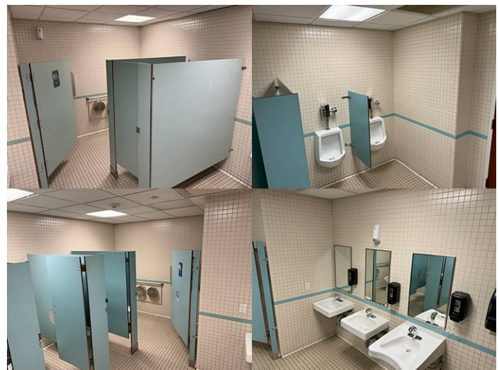
Public Restroom (Typical)
