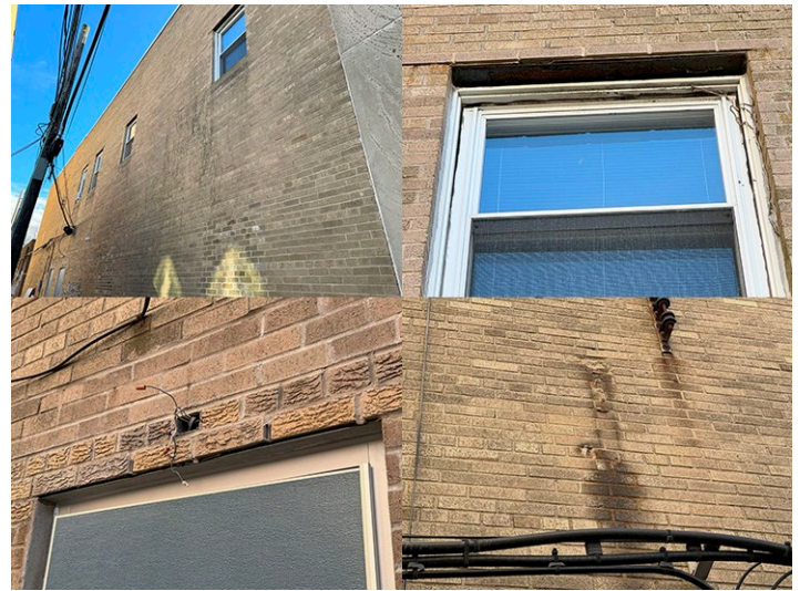
Exterior Masonry Walls – Brick (North Side)
