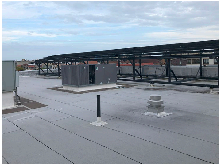
Roofing – “Built-Up” System
