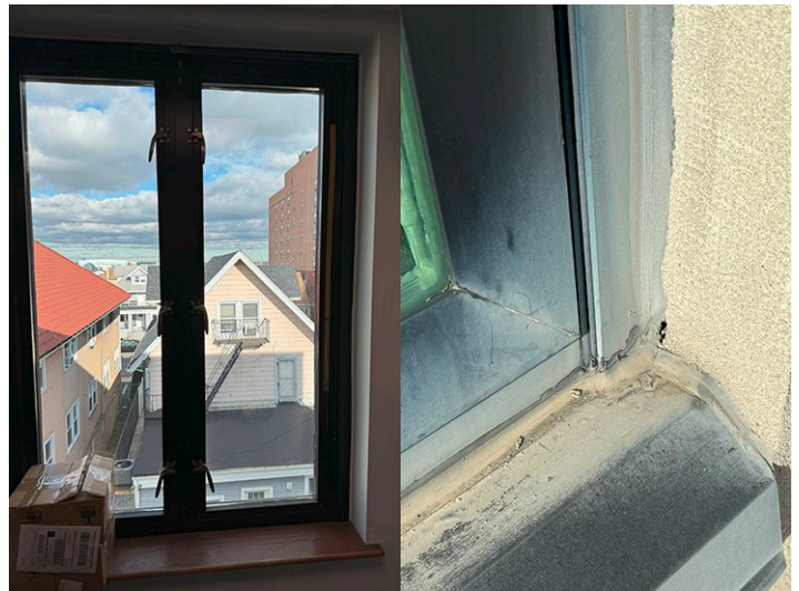
Window System - Operable 1997 (3 rd Floor)
