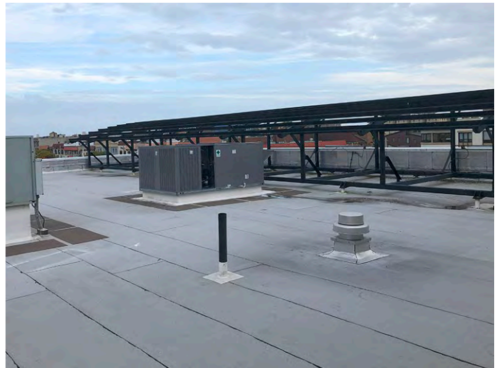
Roofing – “Built-Up” System
