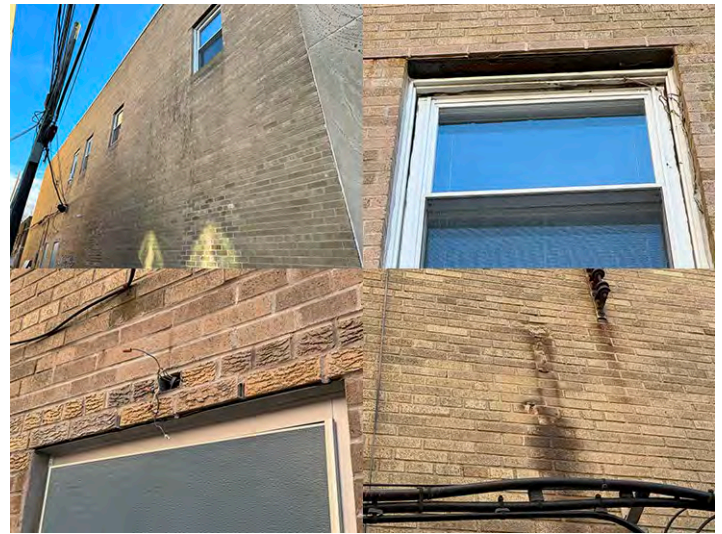
Exterior Masonry Walls – Brick (North Side)
