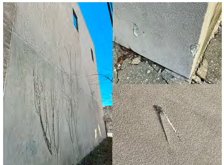
Exterior Wall – EIFS System
