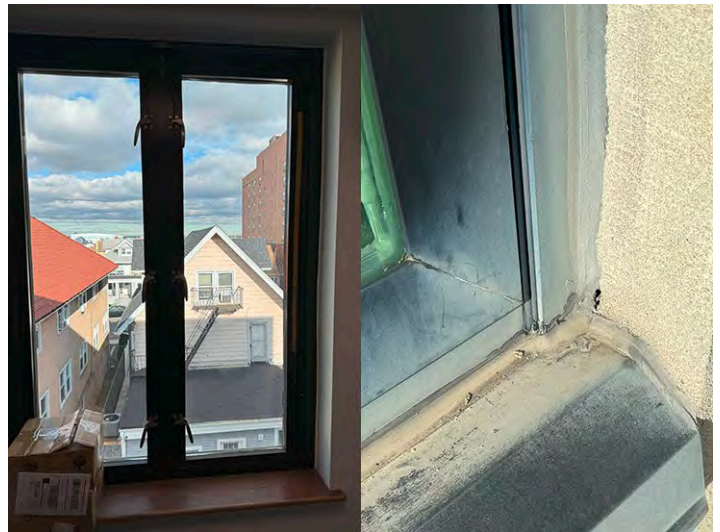
Window System - Operable 1997 (3 rd Floor)
