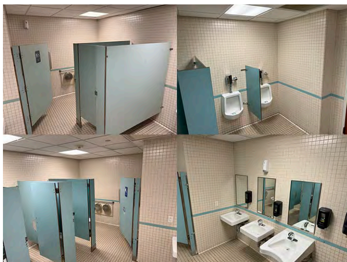
Public Restroom (Typical)
