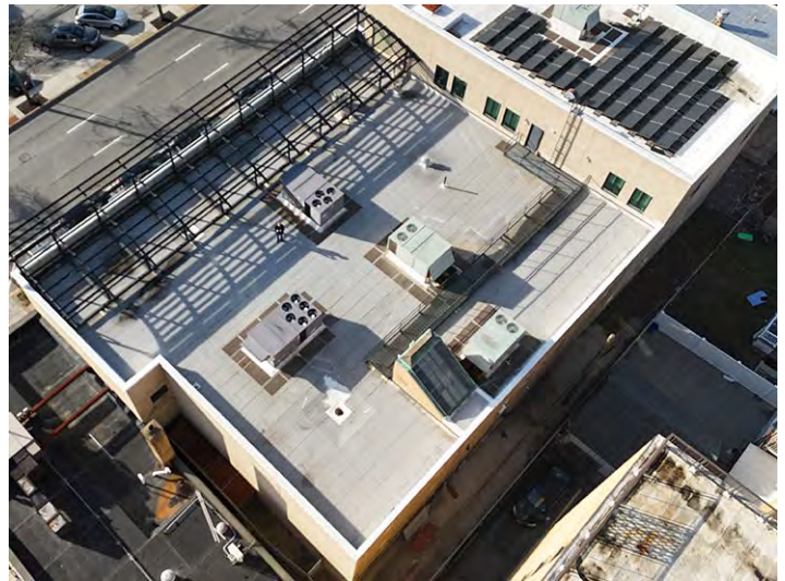
Roof – Lower & Upper
