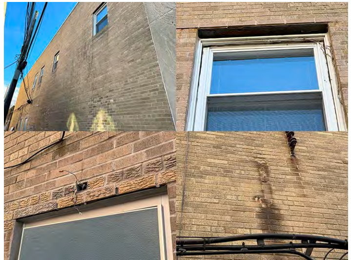
Exterior Masonry Walls – Brick (North Side)
