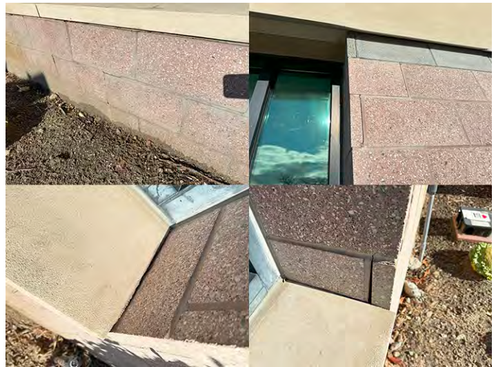
Exterior Masonry Walls – Concrete Block (South Side)
