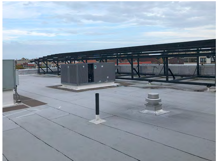
Roofing – “Built-Up” System
